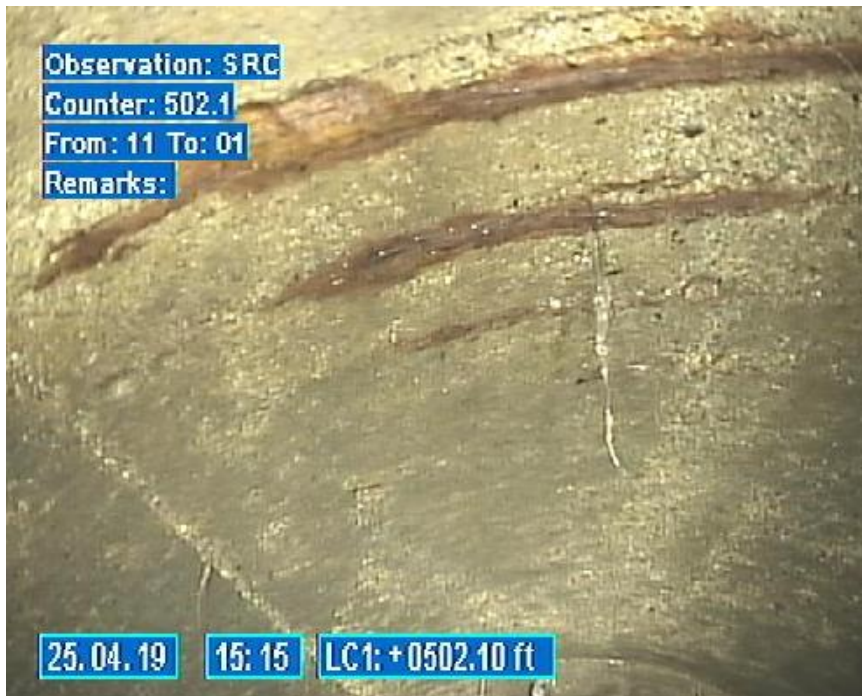
Image at 502.10' shows surface reinforcement.
